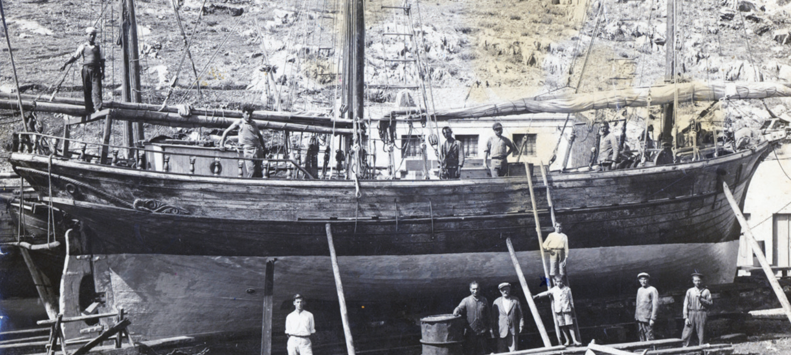
The Anna in dry-dock while she was being fitted with an engine in 1928. Until recently, it was thought that this photo was taken on Kastellorizo, but further investigation has revealed that the location is in fact the Harani shipyard in Symi.
