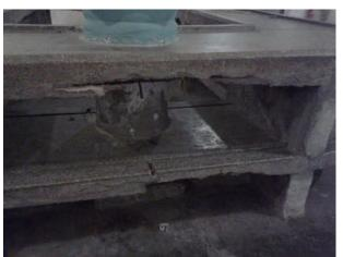
The monument lays deserted without any conservation and is not used anymore as a market place. It is situated on the waterfront and that makes the construction vulnerable to damages due to erosion of the reinforced construction.
