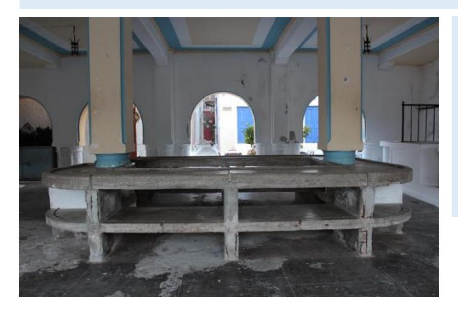
Centrally at the market there is a bench for fish. It is made out of graniglia: one of the first materials that was born thanks to the recycling of waste from the processing of marble and stone, reinforced with cement and steel, colored with natural oxides and mixed with water.
